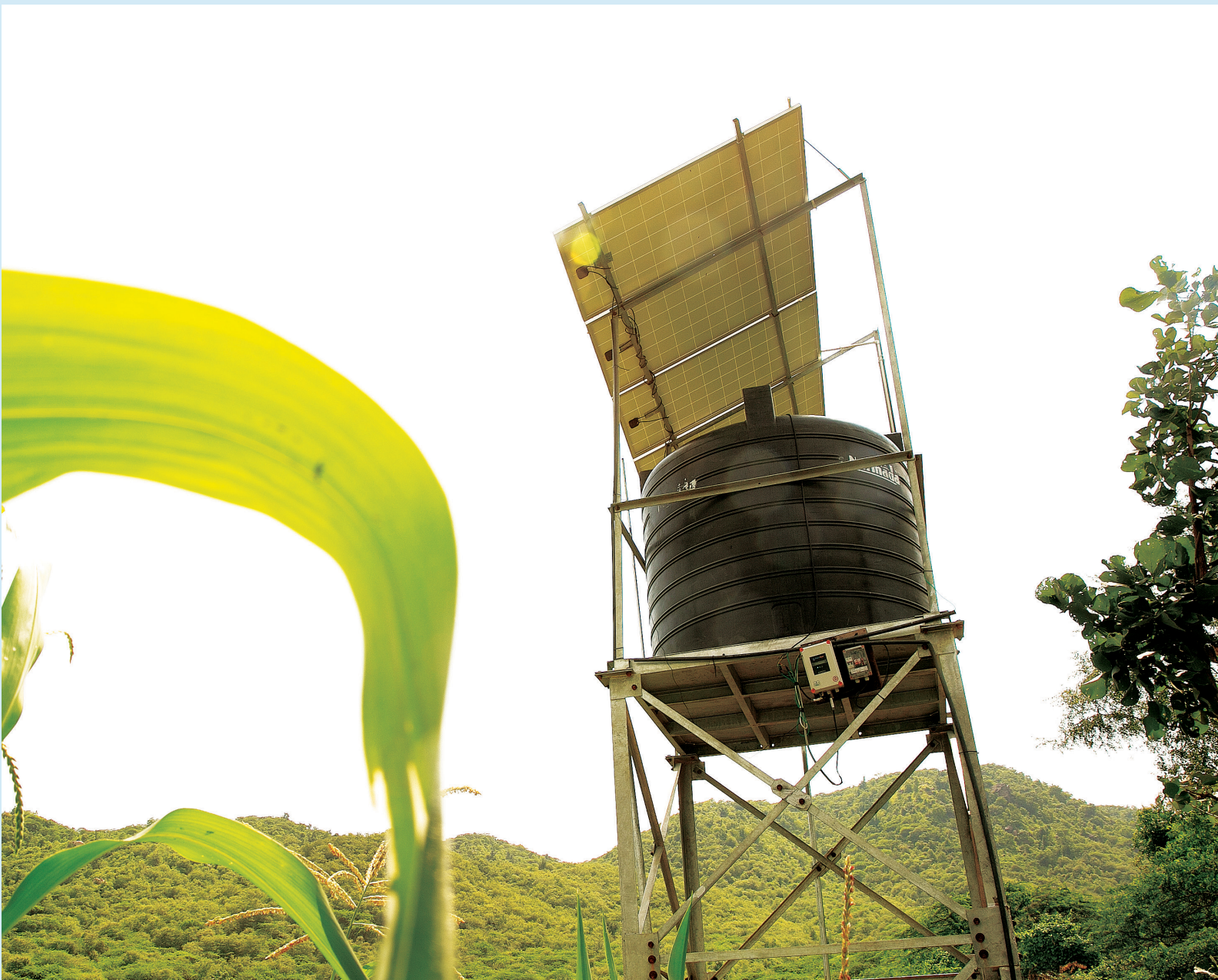
A solar operated water pump in a village in Chhattisgarh
