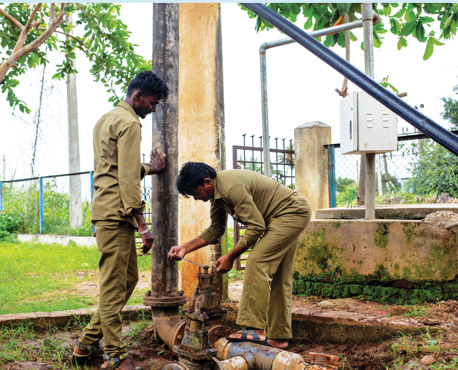
Men fix the outlet valves of the Overhead Tanks in Bennihalli village, Gadag district, Karnataka
