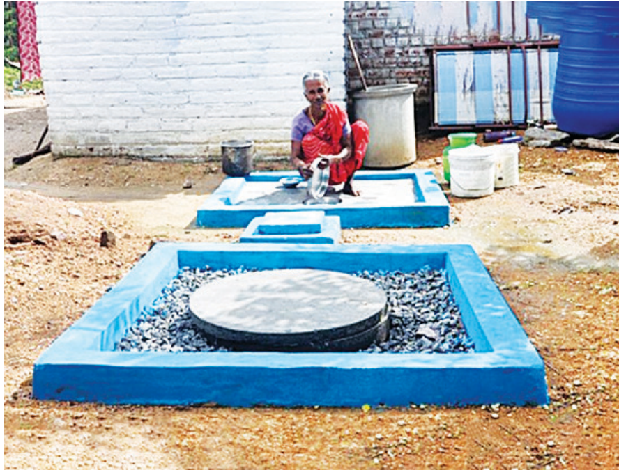
Soak pits for greywater management in a village in Tamil Nadu
