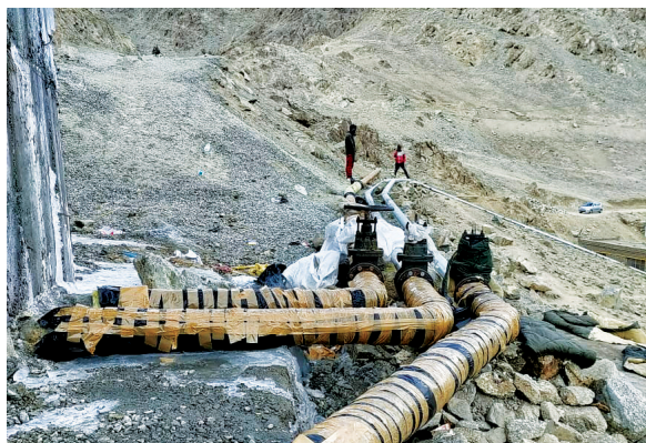
Insulated water supply pipelines
