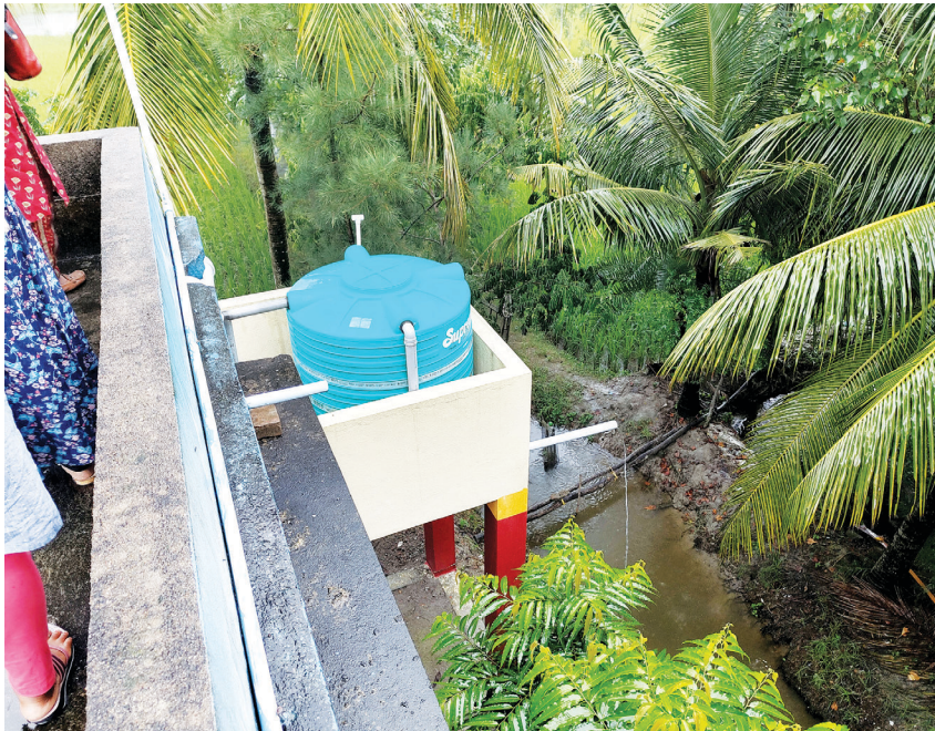
Rainwater harvesting system in a rural household in West Bengal
