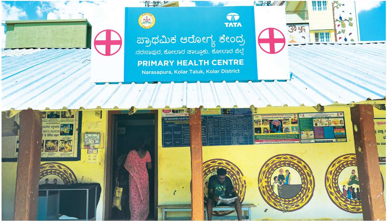
A DiNC-enabled Primary Health Centre in Narasapura, Kolar
